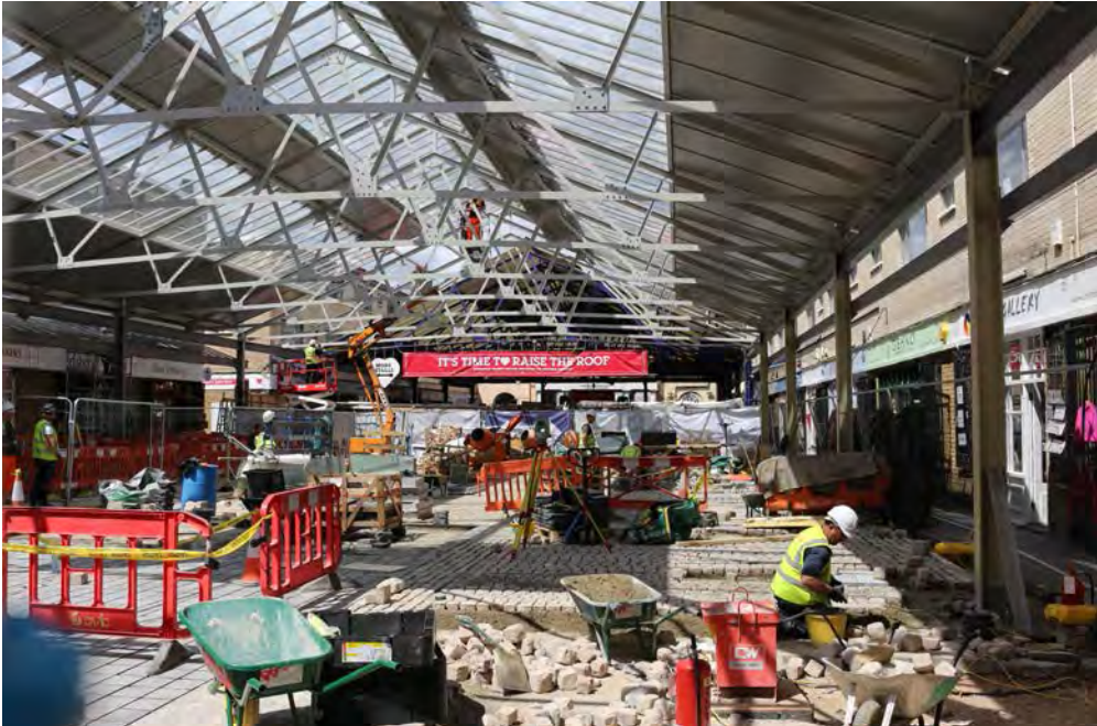
Greenwich Market Restoration – Phase II, 2015
