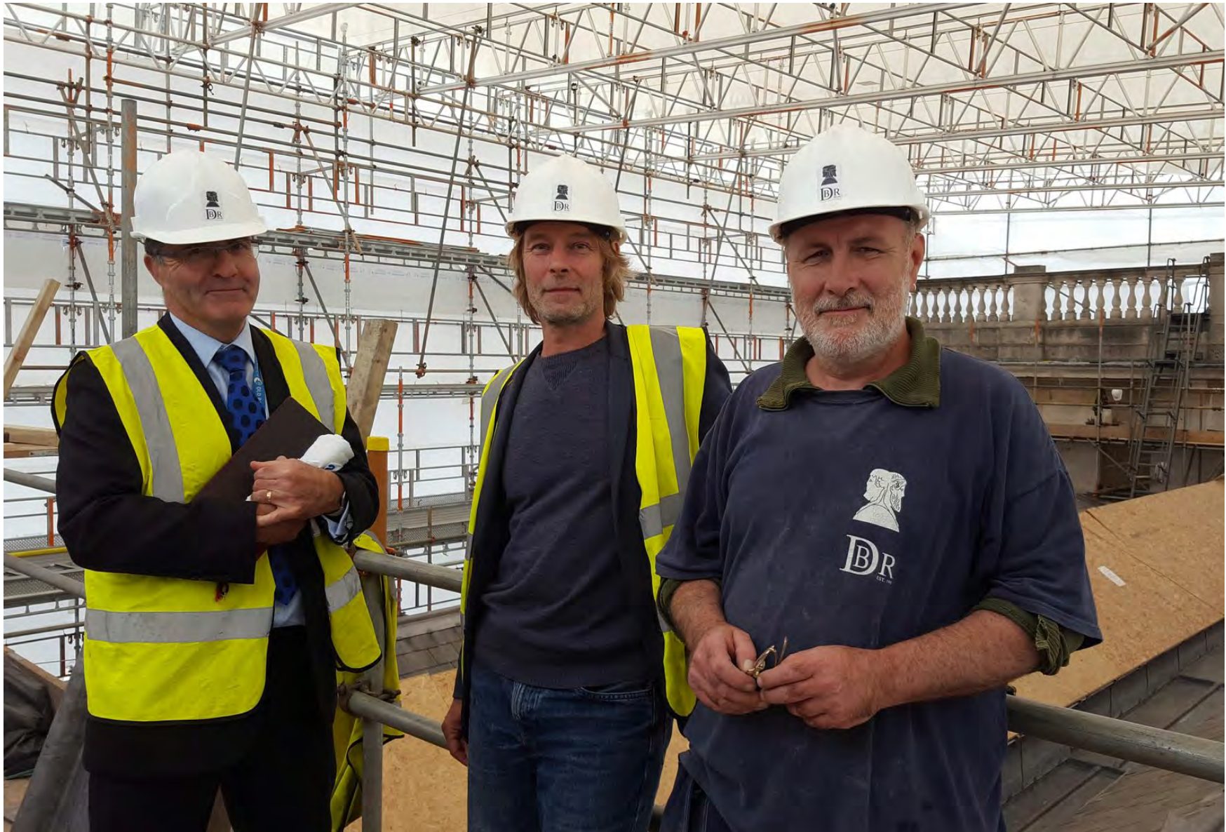
Conservation work in progress, King William Court roof – May, 2016
